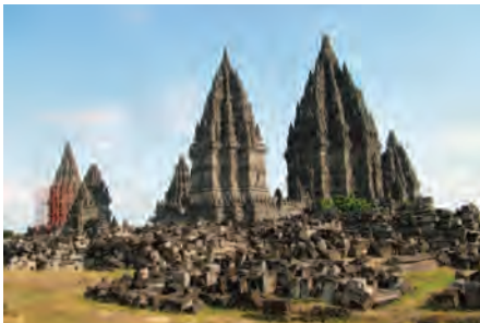
Earthquake damage at Prambanan
